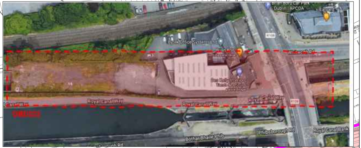
AERIAL PHOTO TRACK LOWERING PHOTO 1
